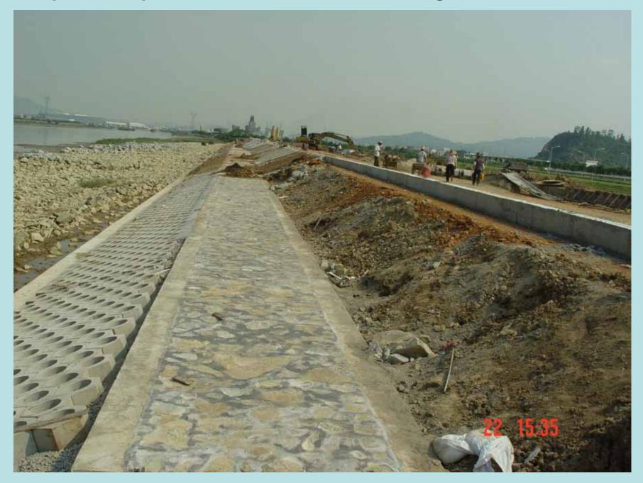
Both sections were paved with hollow bricks with 25 cm diameter holes. One set is 10 cm deep and the other 25 cm
