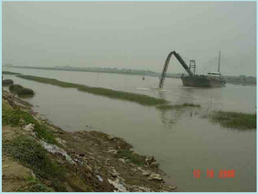
First the slope of the embankment was reshaped, the mud flat covered with riprap rock and the slope with hollow bricks
